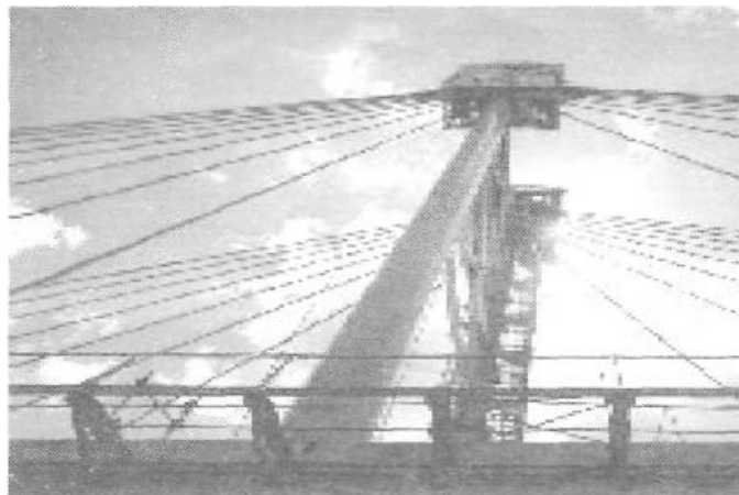
The Nelson Mandela Bridge
