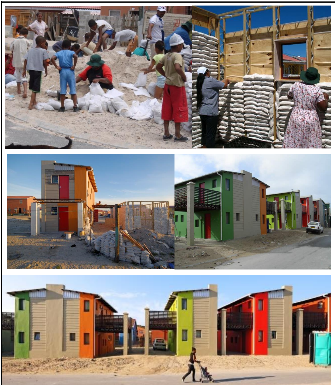
FIGURE 1: 10x10 Low Cost Houses , Freedom Park in Mitchells Plein, Cape Town, by MMA Architects.
