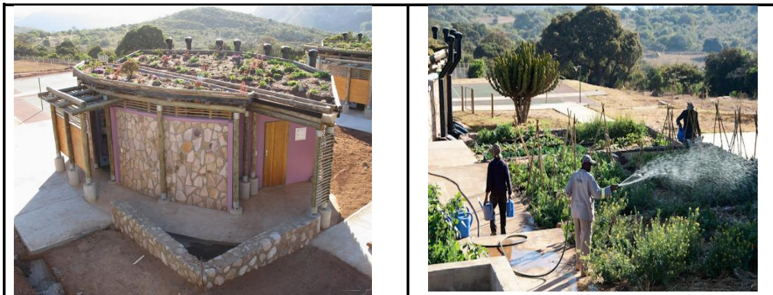
Toilet block: Toilets use a dry composting system which is removed by the education dept. A roof garden acts as insulation.
